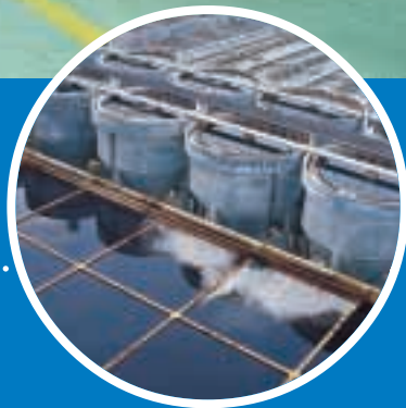
Sewage Treatment Plant
